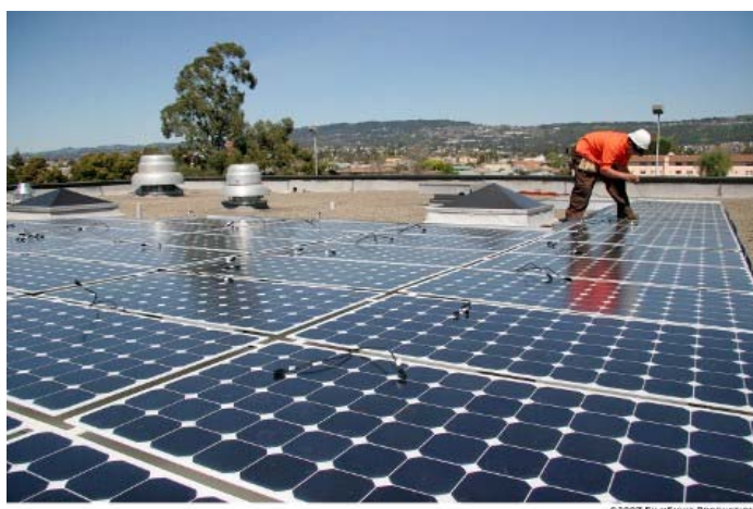
Installation of solar photovoltaic panels (Source: AC Transit)
