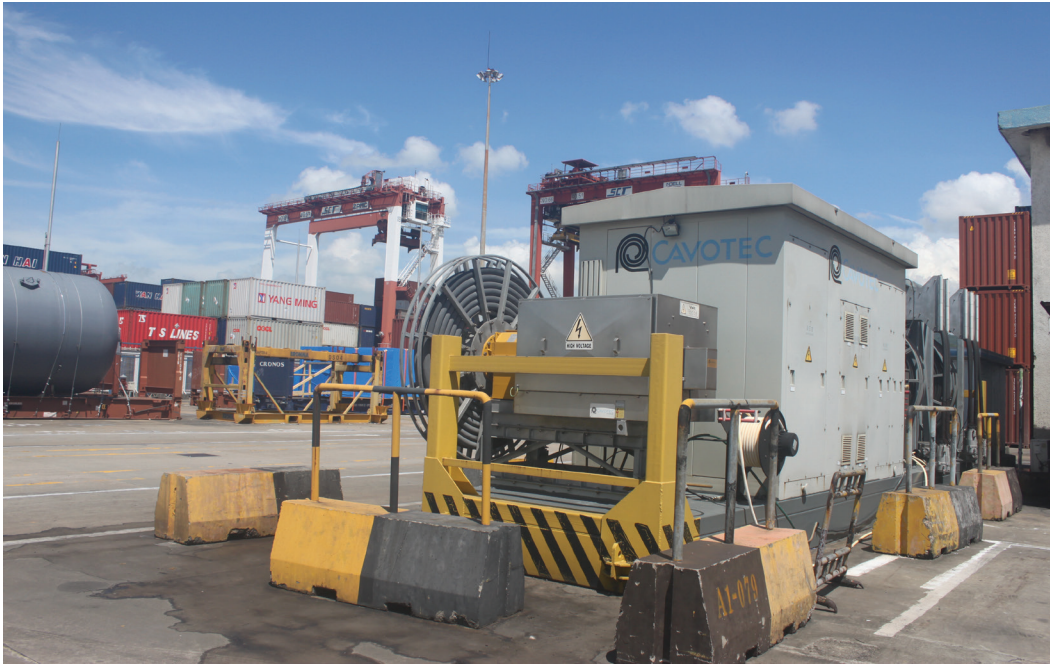
Figure 2. An example of shoreside shore power infrastructure in Shekou.
