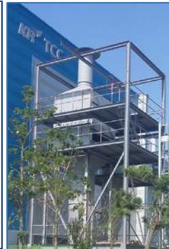
❖ Installation and proof of SO<sub>x</sub> scrubber for ships toward IMO global sulfur cap (2018~2021, Ministry of Oceans and Fisheries)
