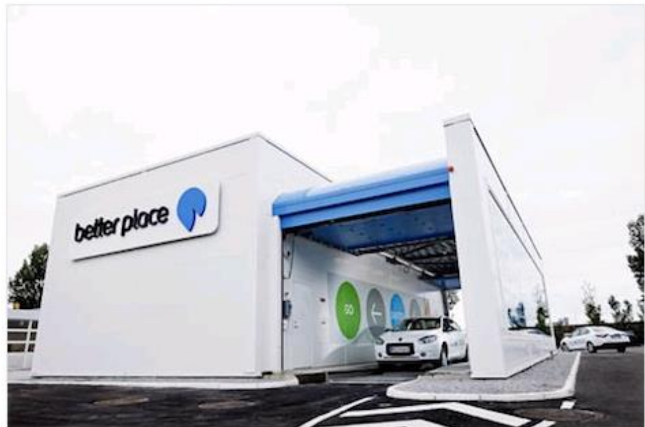
Figure 20 Example of a battery swapping station from Better Place
