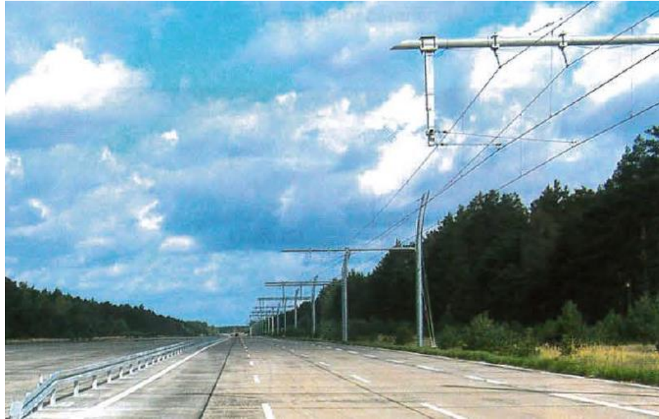
Figure 21 Catenary for hybrid-electric trucks
