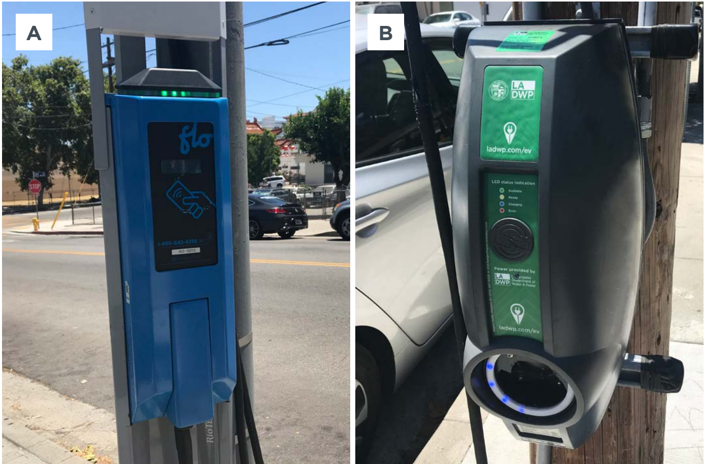
Figure A-1. A Flo streetlight charger (A) and LADWP's power pole charger (B) in Chinatown, Los Angeles. Photos taken by Anh Bui, ICCT.
