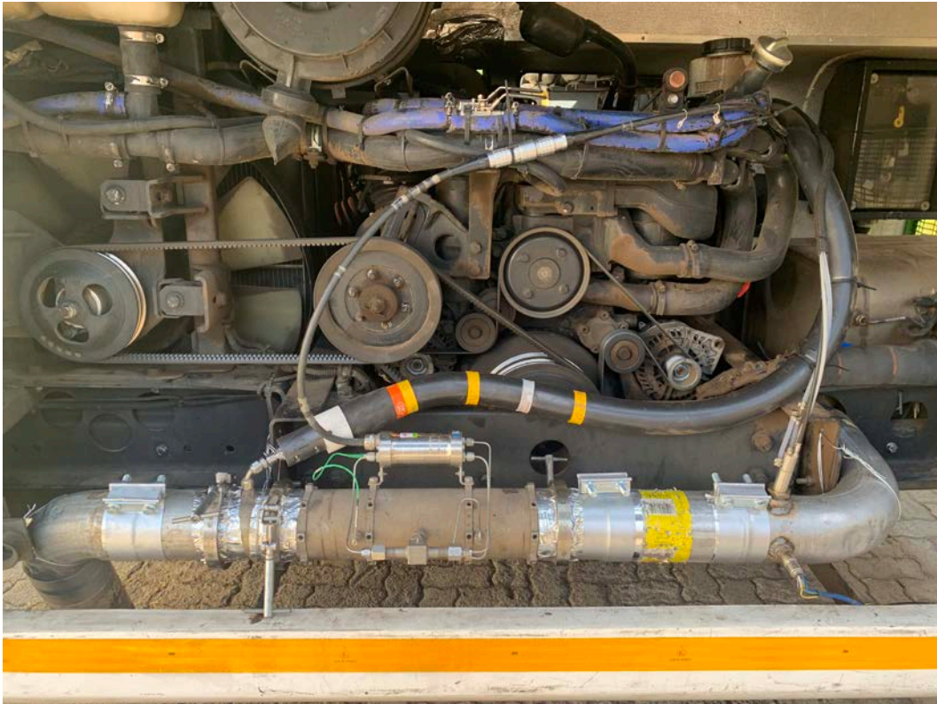
Figure 7. EFM and sampling line installed in the back of Metrobus bus # 2097. Source: WVU
